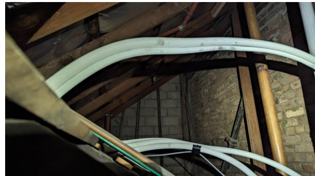
Figure 2. Skillion roof extension fixed to wall of 300GS
