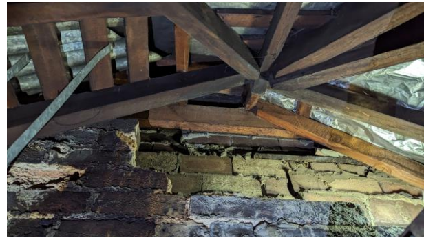
Figure 4. Apex of roof supported off 300GS façade wall
