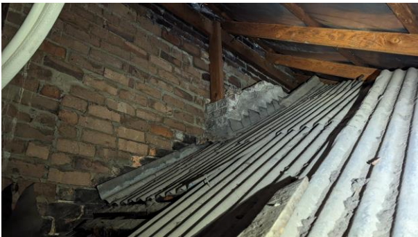
Figure 1. Earlier roof sheeting with skillion roof over
